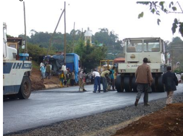
Surfacing the new road by the hospital.
