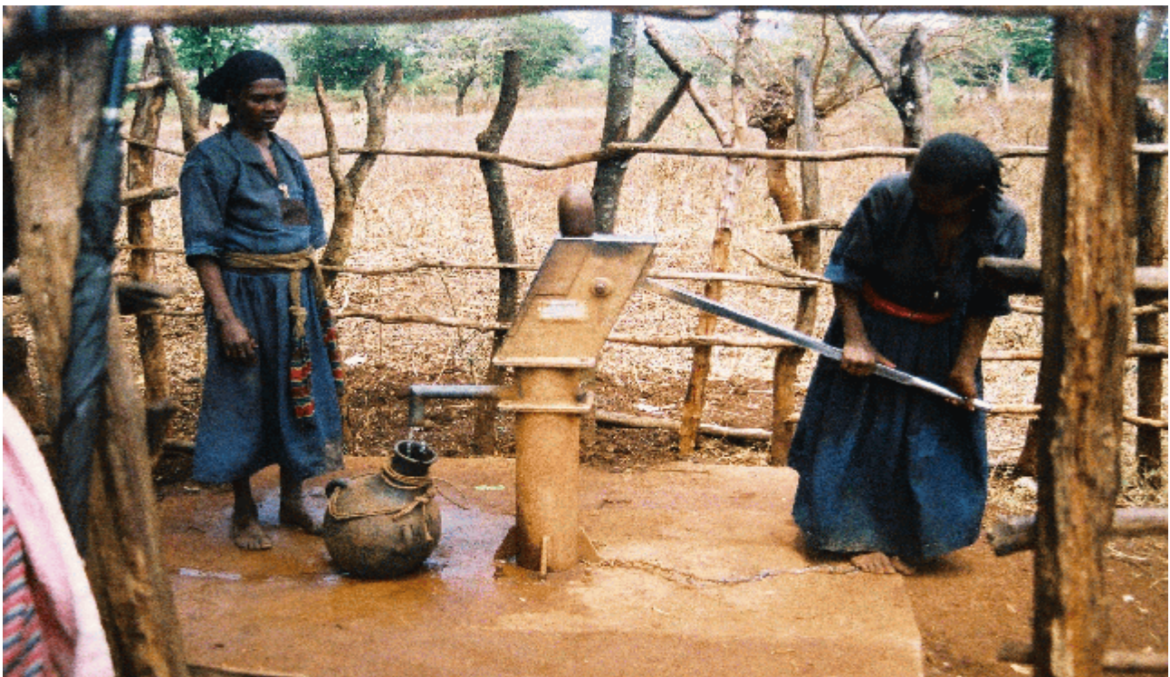
Refurbished deep bored well in the Wama Valley near Nekemte.
