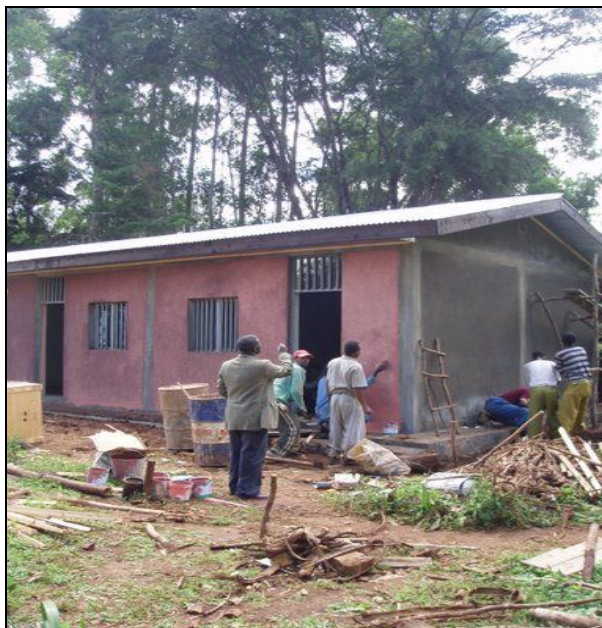
Qes Alemu Nega checks work on the spectacle workshop
